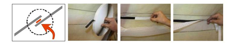
• Surfaces must be dry and free of release agents like grease, oil, tensides, dirt and dust.
